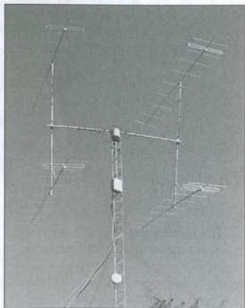
LU1CGB Yaqi system for 144 MHz on Jan 30 th
